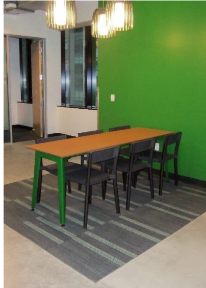
Carpet Example 22 Carpet tile as area rug with standard resilient edge guard.
